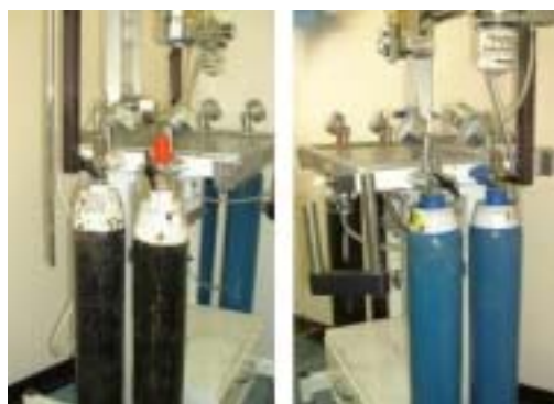
Figure 1. Gas Cylinders – Oxygen (on the left) is presented in black and white cylinders; Nitrous Oxide (on the right) in blue cylinders.
